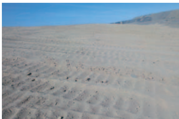
Preparation of topsoil stockpile for vegetation
